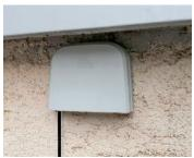
The Eline® OTB enables an optical transition between an outdoor drop cable and an indoor subscriber cable. The OTB can also be used to realize a repair between two drop cables, up to 4FO.
